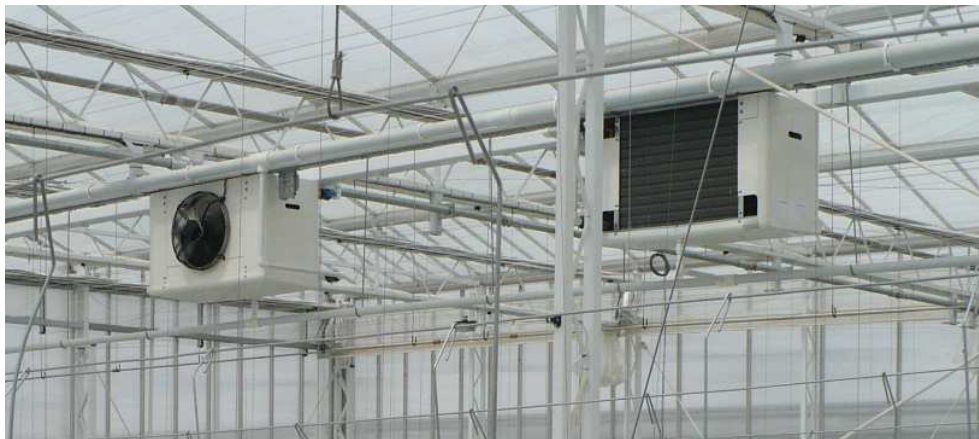
Figure 15. Picture of two of the six air conditioners in the 'Sunergy Greenhouse'. The left-side heat exchanger demonstrates the fan for air flow and the right one shows the heat exchanger surface on the suction side. The coolers are mounted at 6.5 meters height.
