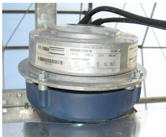
Figur 6. Detail photo of fan motor of the OPAC 106 heat exchanger
